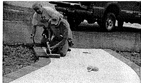
Bob Weyenberg & Roy "Brownie" Brown laying the first brick order in 2008.
